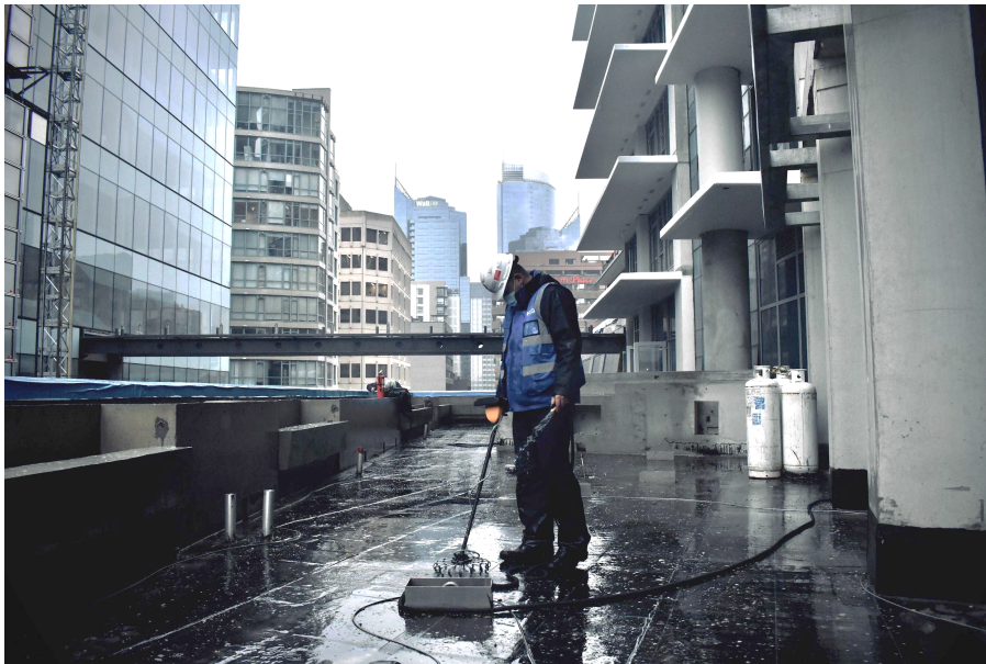
Above: An SMT Technician performs a Digiscan service on an inverted roof membrane
